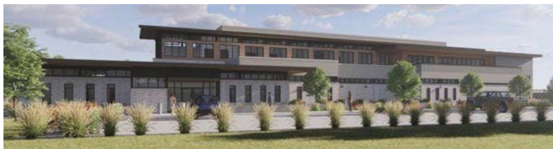
Across the street from a county sheriff's department, Money Metals Depository is by far the largest such facility in the Western U.S.
